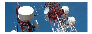
**Cellular networks** use fixed-location transceivers to create 'cells' of wireless coverage over land areas, and relay data via 'handovers' to neighboring cells as users travel into new cell geographies.
